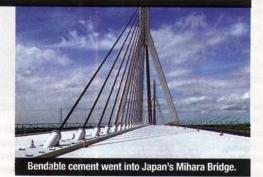
The flexible concrete is three times more expensive than the ordinary kind, but Li says the cost should be offset by fewer repair bills and a longer life span. Because it is 500 times more flexible, Li believes his concrete could
